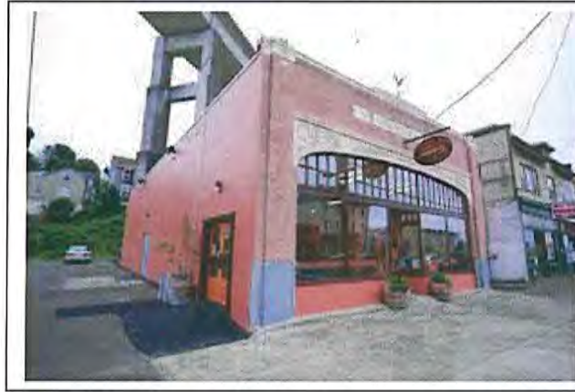
Figure 14.115-5: Non-Industrial Building, Flat Roof Behind Parapet Wall
